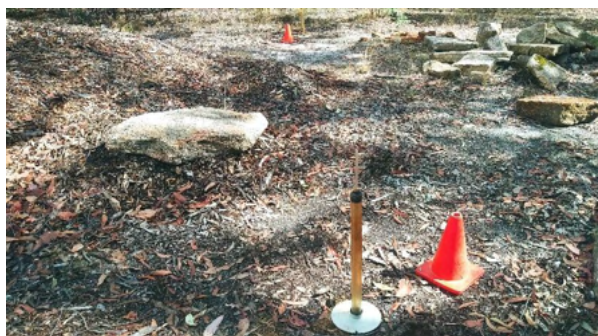
Another view of the LCA test area. Some surface debris, concrete wood pile and some soil piles need to be removed before installation.
