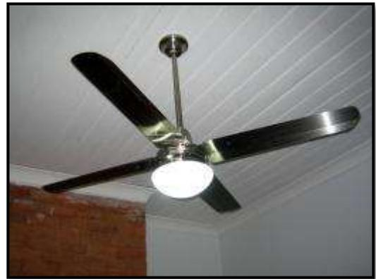
*Figure 6: Install ceiling fans with a summer/winter switch to offer air movement and cooling.*
