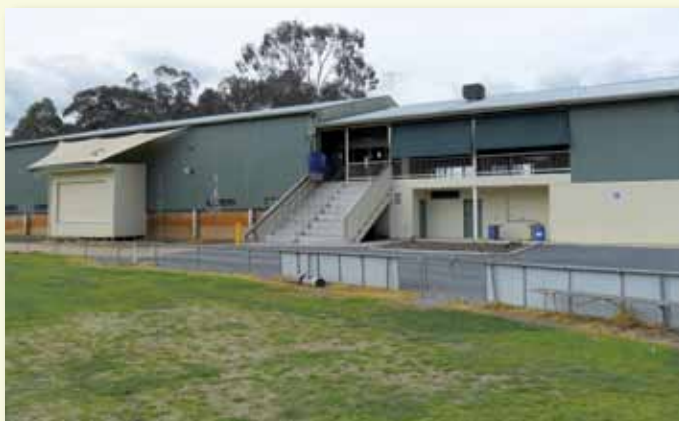
▲ The finished Yackandandah Sports Park Centre.
