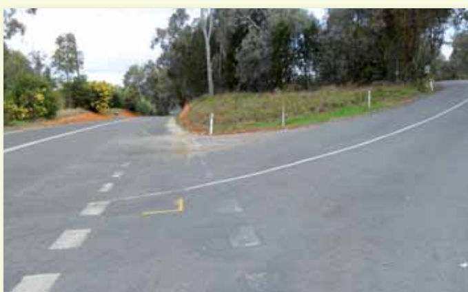
▼ The work upgrading the Back Creek Road / Kirby Flat Road intersection at Yackandandah cost $62,000.
