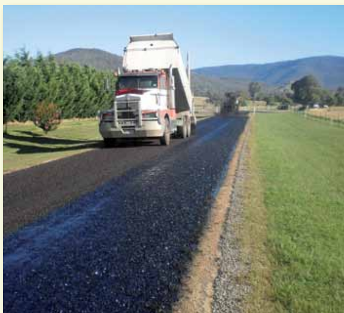
▲ Resealing work on Flynn's Road, Yackandandah.
